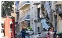
Powerful explosion in central Athens, two-story building collapses and...
