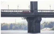
Two Russian drones strike Pivdennyi Bridge in Kyiv, public transport temporary...
