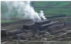
Albchrome poisoned Elbasan with hazardous waste, 320 tonnes of toxi...
